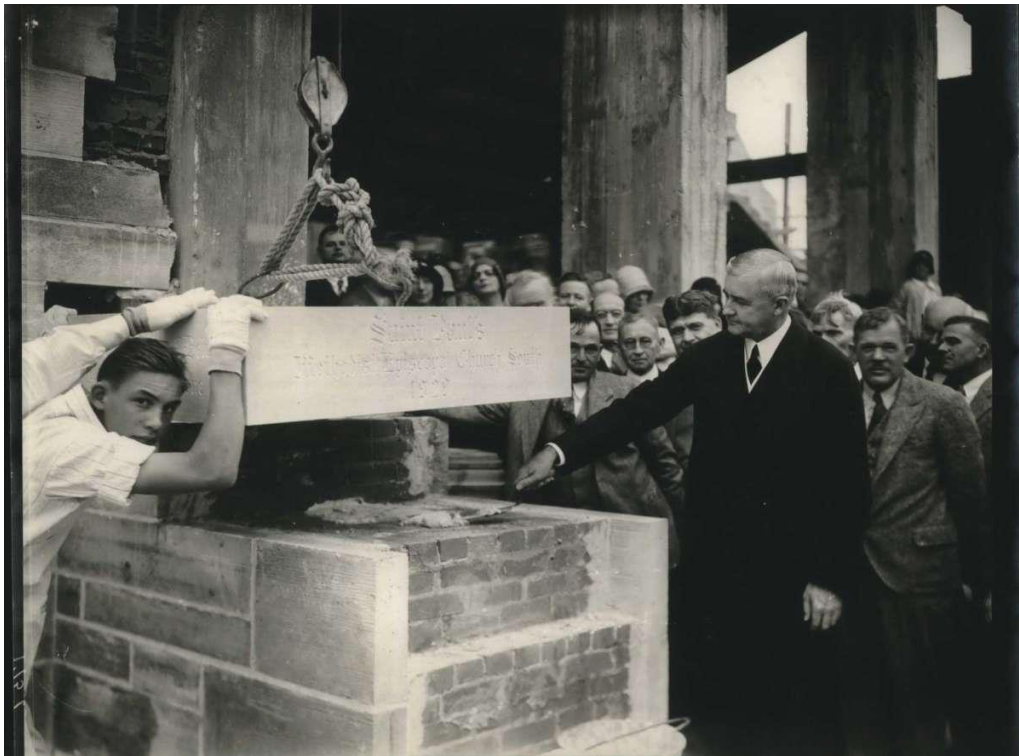
Laying of the corner stone at St. Paul's Methodist Church dedication by Jesse H. Jones, Houston, Texas.
