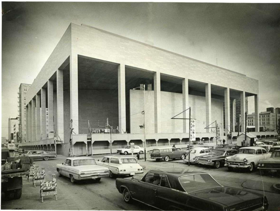
Jones Hall under construction in 1965. For more vintage photos, scroll through the gallery. Curtis McGee/Houston Chronicle
